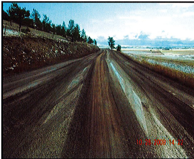
Photo 4: The width of the gravel road can vary depending on gravel displacement. Cut and fill slopes are steep relative to the proximity of the driver.
