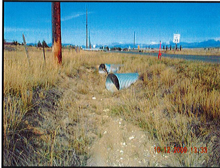
Photo 6: Double culverts installed just south of the Helena Valley Canal, MP 1.6.
