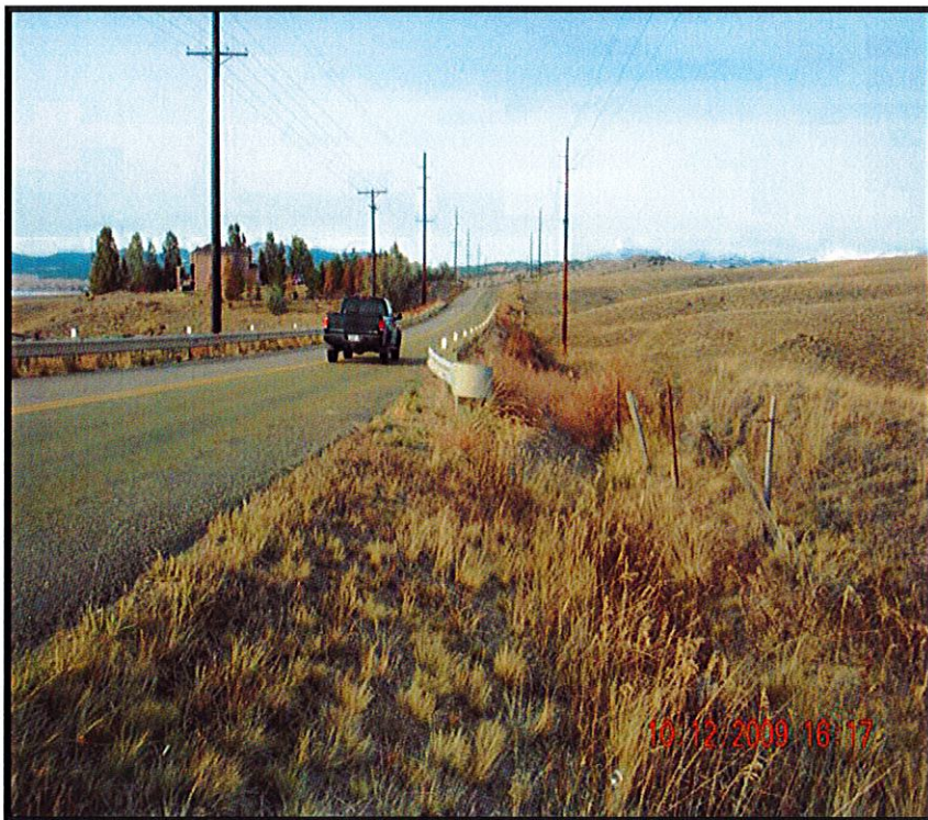
Photo 3: Photo of a cut section transitioning to a fill section through a drainage. Note the guardrail installed for safety. Roadside slopes are steepened to fit within utility and right-of-way limitations.
