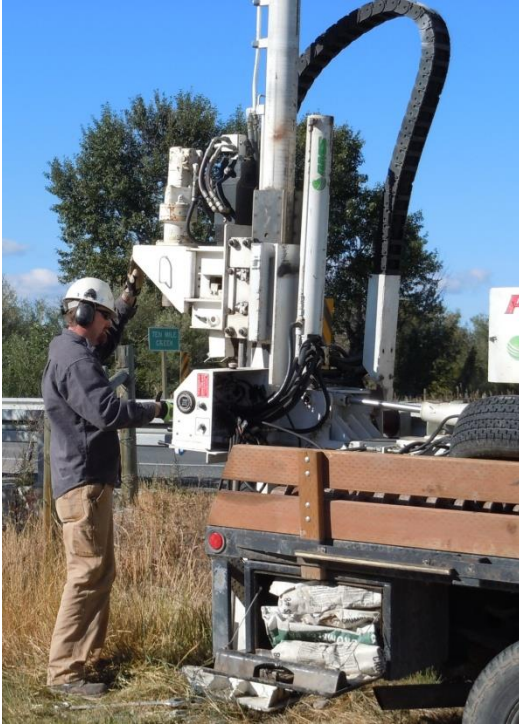
Figure 4-1 Piezometer Installation
