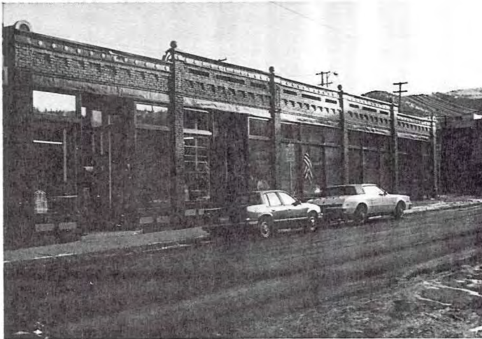
(Left Below) The C.W. Cannon Building after rehabilitation. Original sized windows are restored complete with transoms. The brick facade has been cleaned and painted. Decorative features of the building cornice have been emphasized by the creative use of color. Bright afternoon sunlight is controlled by mini-blinds. The storefront rhythm is restored without altering the interior use.
