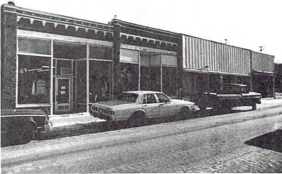
(Left Above) The C.W. Cannon Building before rehabilitation. The far right bay of the building had been "modernized" with a sheet metal false front. The rhythm of the building facade was disrupted and many historical details lost. Transoms were covered, permanently restricting the natural light.
