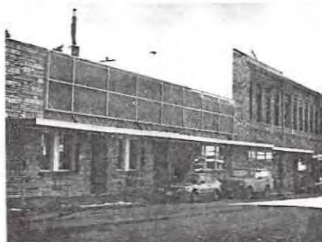
(Left) Vertical awnings became rare as the style shifted to the horizontal. Fixed canopies were used to emphasize this line. The second stories of these old buildings were neglected and attempts were made to hide them beneath the new facade facing.
