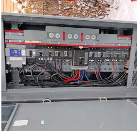
Load fed from buss along bottom
