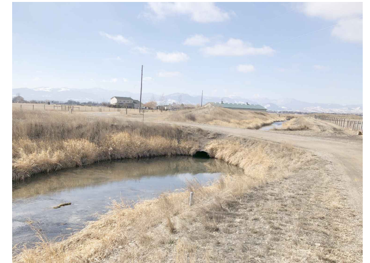
VIEW OF EXISTING CULVERT - LOOKING SW
