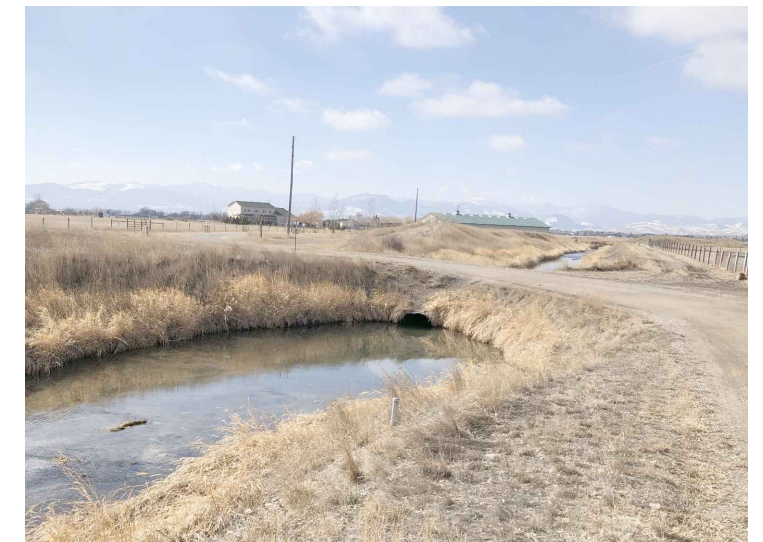
VIEW OF EXISTING CULVERT - LOOKING SW
