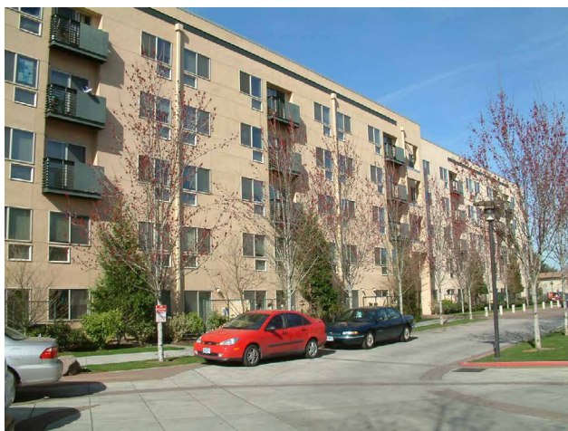
Center Commons, a transit-oriented development in Portland. Planners provided fewer parking spaces than apartments, so residents illegally park their cars in a fire lane or on the sidewalk.
