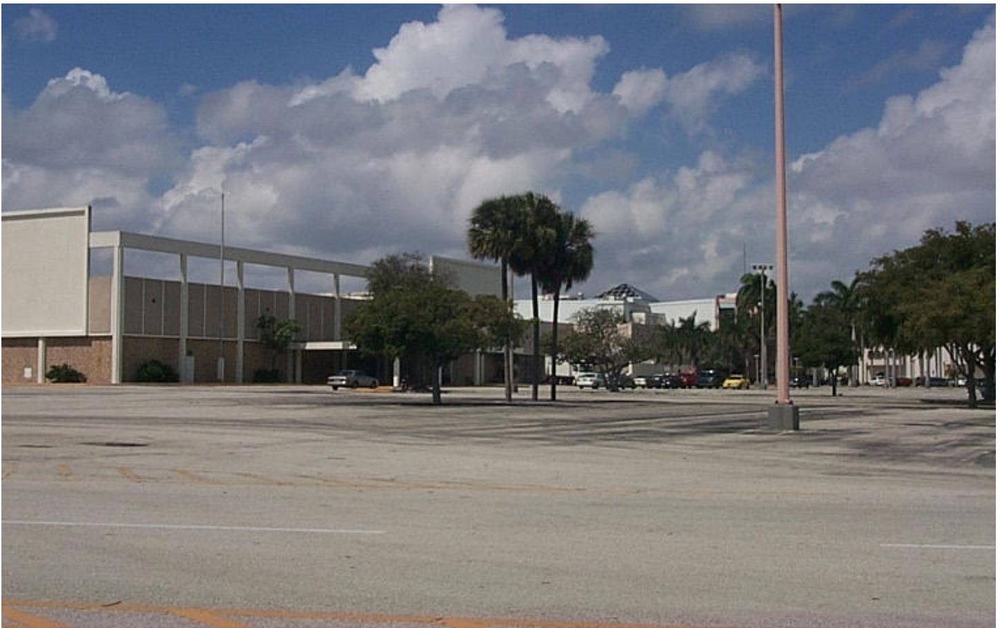
This mall, Pompano Fashion Square in Pompano Beach, Florida, is a good example of a parking lot that could be repurposed for green infrastructure.
