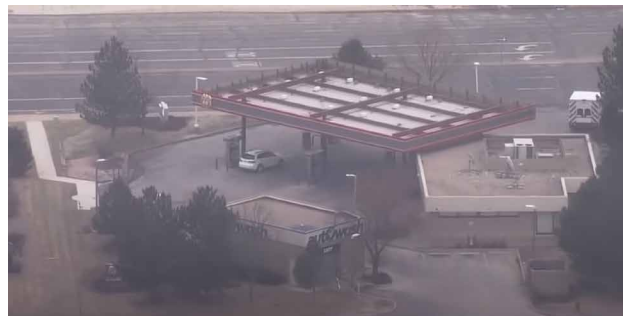
This gasoline station survived while nearby homes did not, demonstrating the value of firewise design.
