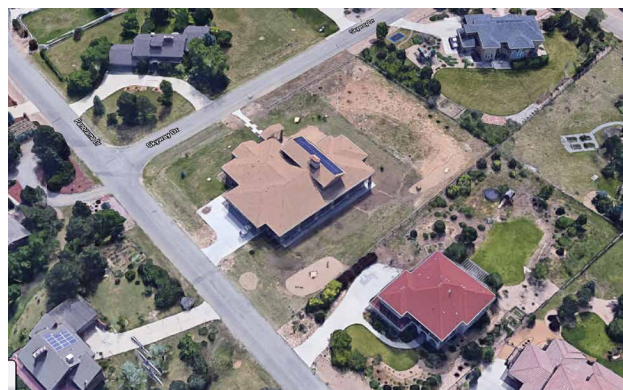
The center home in this photo was the newest in the neighborhood and was saved by the fact that the owners had not yet grown or installed any trees or shrubbery. All of its neighbors shown in this photo burned to the ground.
