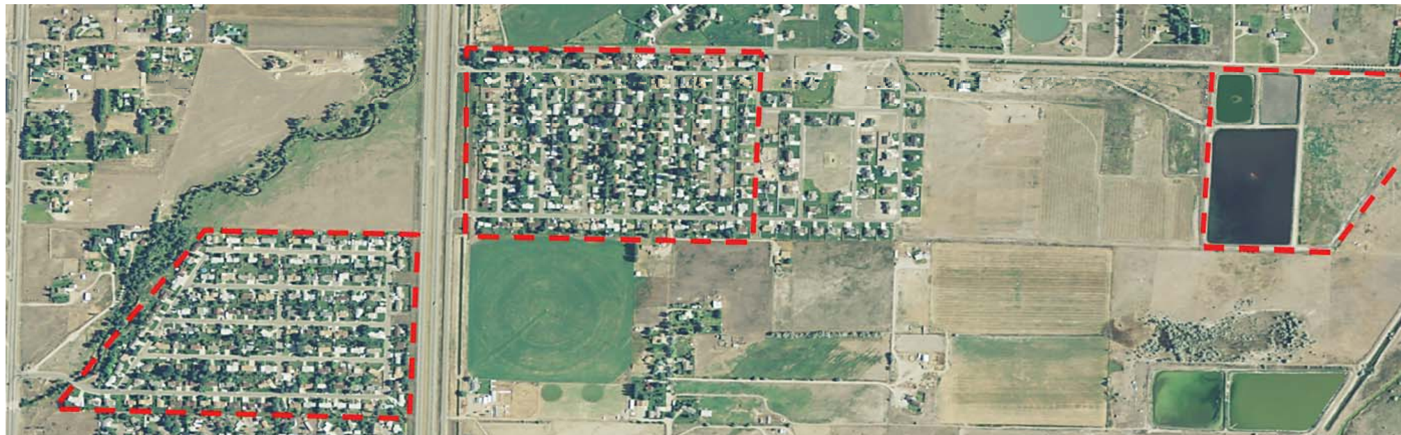
CH 3 FIGURE 2— Massive failure of the Ten Mile Creek/Pleasant Valley Estates sewer lagoons led to lawsuits and a $5.5 million dollar system fix.
